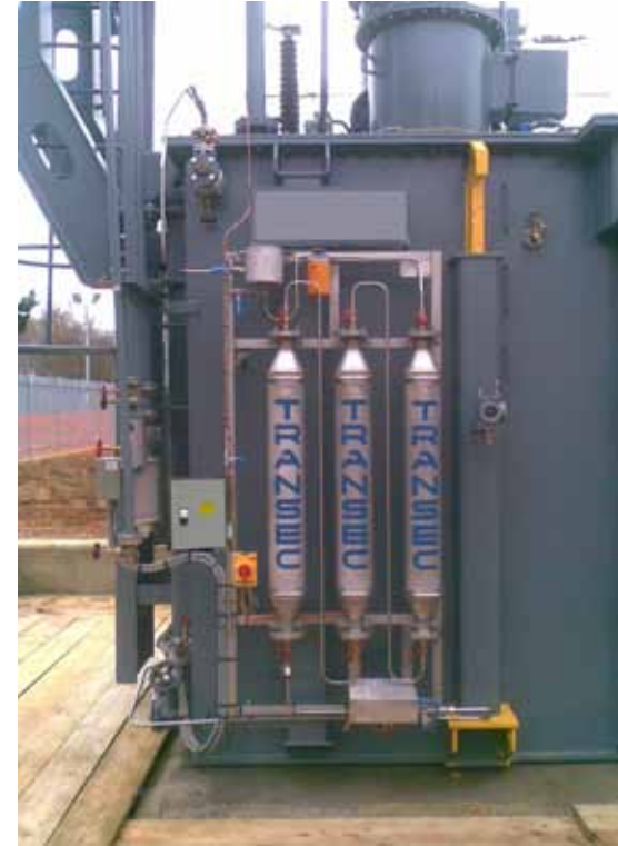
A TRANSEC Unit consists of one or three series-connected cylinders. Each on-line transformer drying unit continuously removes water from oil in generator, transmission and distribution transformers.
